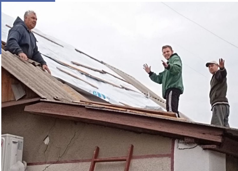
Rebuilding damaged houses in de-occupied territories
